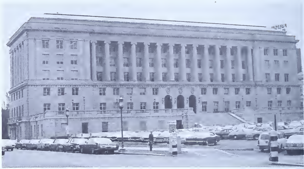
South Office Building, north elevation.
